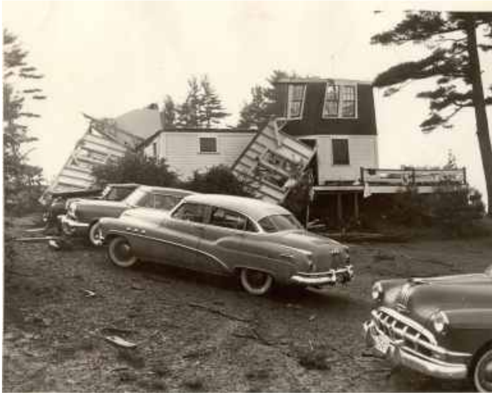
Photo of the tornado damaged remnants of the Exeter Country Club (Courtesy of the Exeter Historical Society)
