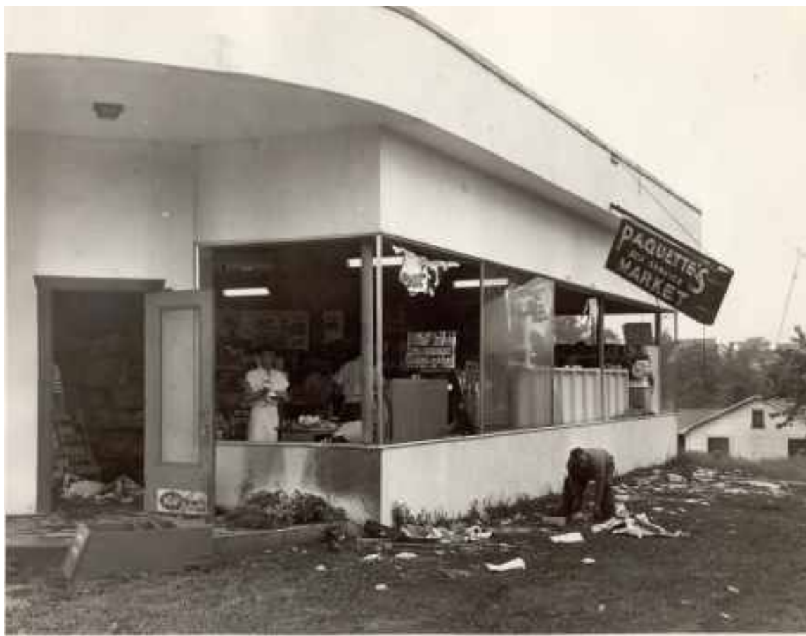
Photo of the damaged Paquette's Market with cleanup in progress (Courtesy of Exeter Historical Society)
